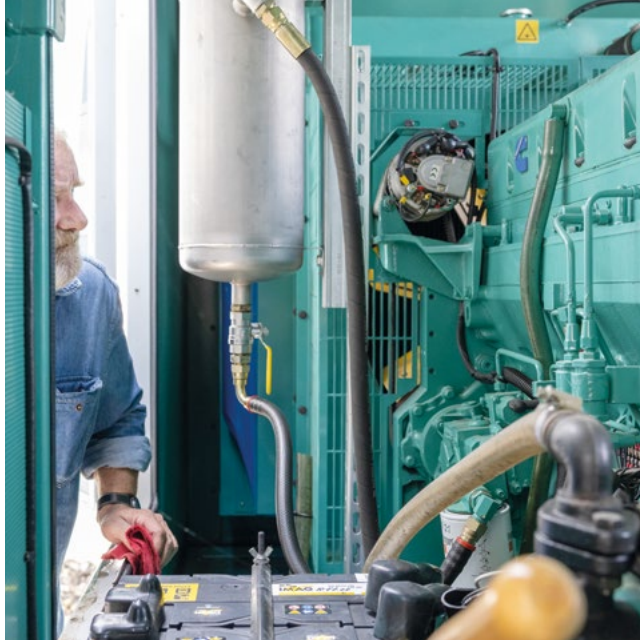
The functioning of the diesel-powered emergency power system is tested monthly.
